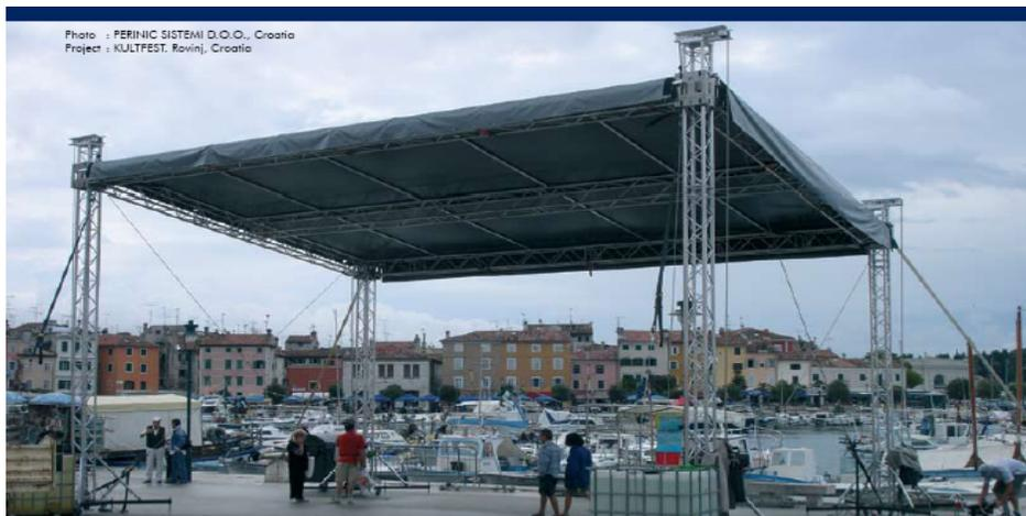
The Flat roof is a tower-based structure with a sloping roof, which is very easy to build. The roof slopes downward to the back of the stage.
